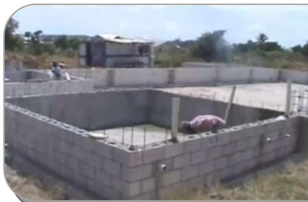
Foundation as at Monday 23 February 2015.
