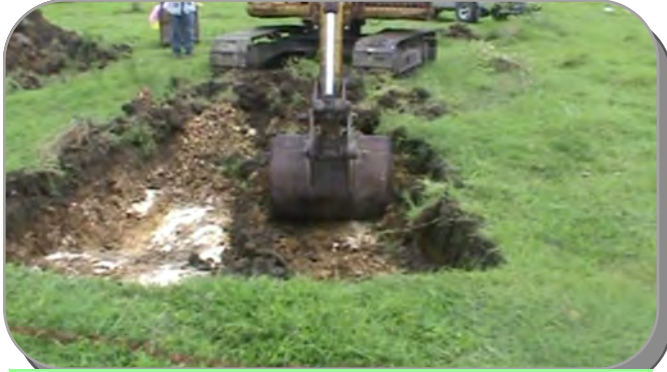
Excavation of Foundation commenced on 24th August 2014
