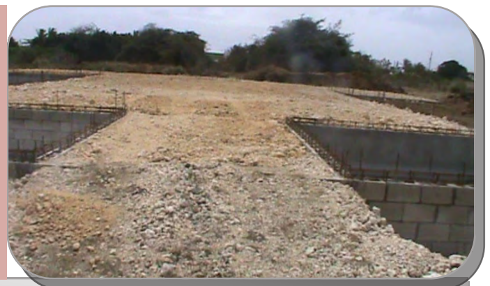
Foundation currently filled with Marl.
